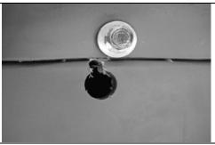
9) Drill out dimples on **inside** of base runners in **rear** (1left runner & 1 right runner) using a 1/2" dia. drill bit. Drill directly on top of 1/2" hole using 3/16" drill bit & 3/16" hole should be open into 1/2" hole. Base PN 19015(roto-mold).
